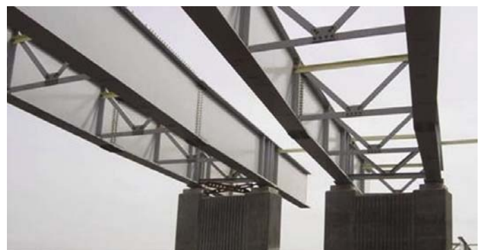
Fig.9: A pair of braced beams.
