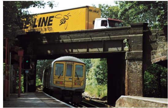
Fig. 3: Over-bridge at Hackbridge, UK
